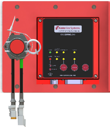
SA1 Control Panel and EMR
